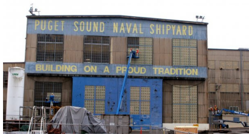
Building 460 before abatement of exterior asbestos & lead
