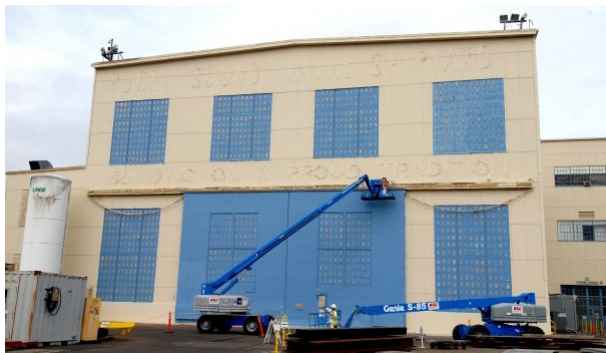
Applying T-B-C to the Transite Siding
