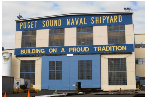
Building 460 after abatement of lead-based paint and asbestos siding
