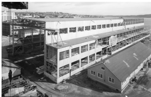
Building 460 during construction - March 5, 1941
